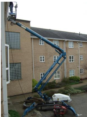
Wall stain cleaning in progress
