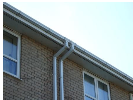
Gutters have now been unblocked and washed
