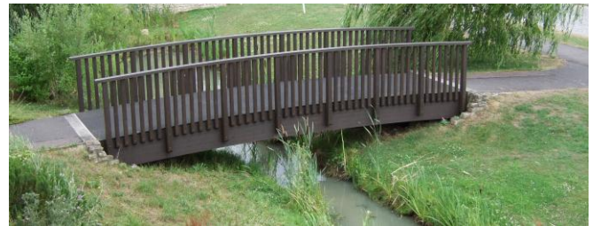
Footbridge looking good after free repaint
